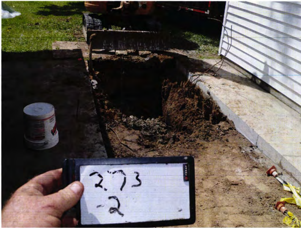
Picture 5: Excavation site of UST 273Birch-2.
