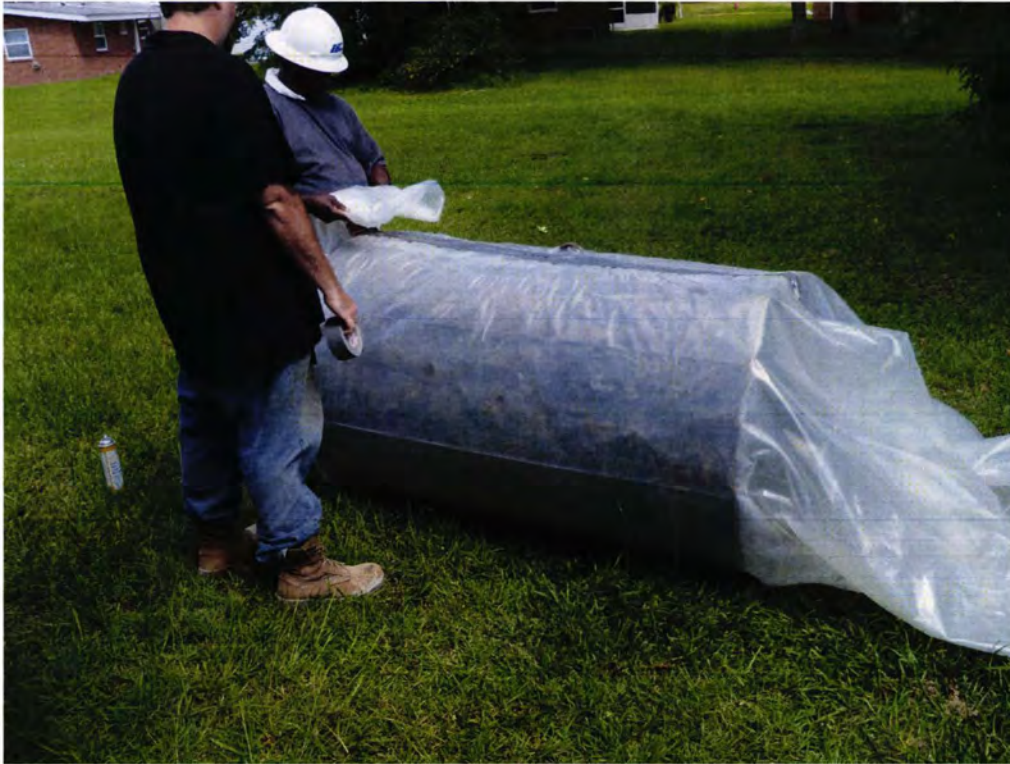
Picture 3: UST 273Birch-1 being wrapped for transport.
