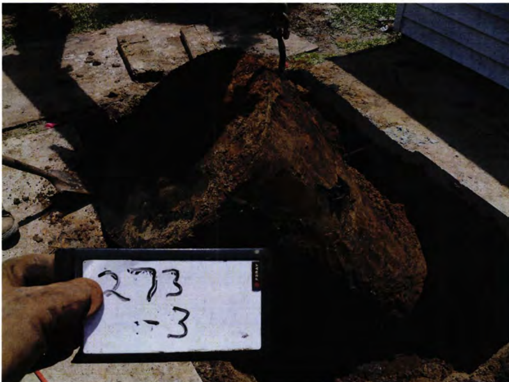
Picture 6: Removal of UST 273Birch-3.
